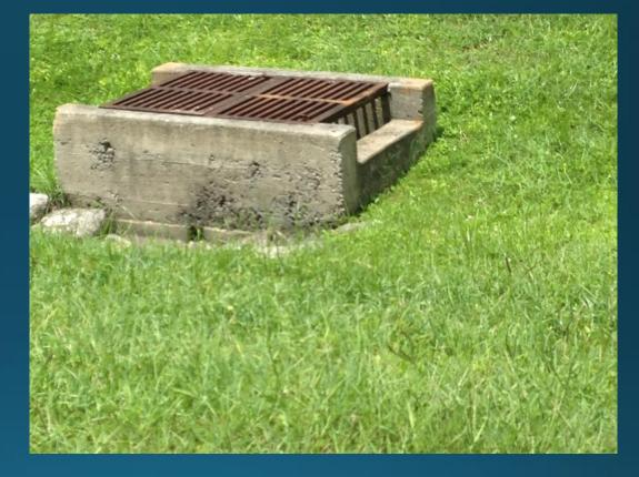
Bonita Springs Swale Box Drain
